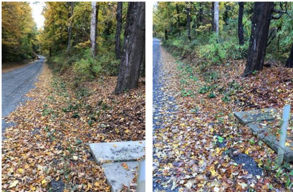
*Figure 13. Photos taken looking uphill of drop inlet (#14) pre-rainfall event (left) and post-rainfall event (right) on Pixley Hill Road in West Stockbridge during field investigations on October 13-14, 2022.*
