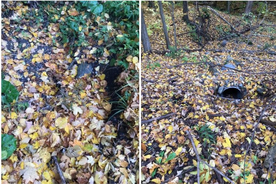
*Figure 6. Condition of the drop inlet (left) and outlet (right) of a cross culvert of a 1.5 ft circular PVC pipe. The pipe is partially deformed and blocked by debris.*
