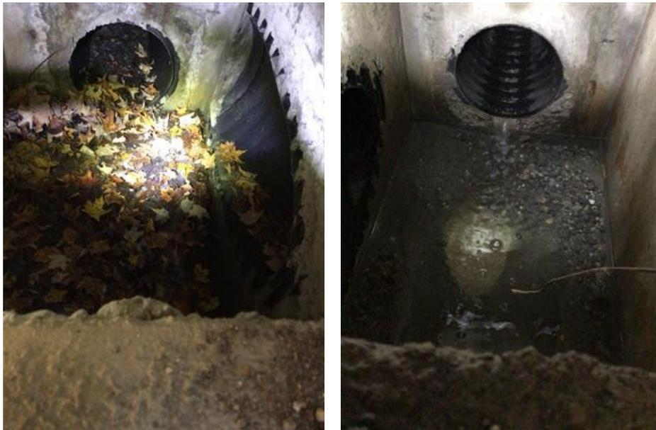
*Figure 12. Photos taken inside of a drop inlet (#14) pre-rainfall event (left) and post-rainfall event (right) on Pixley Hill Road in West Stockbridge during field investigations on October 13-14, 2022.*
