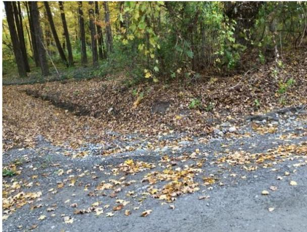
*Figure 5. Condition of the southern portion of Maple Hill Road where culverts have not yet been installed and there is significant flow into the woods, eroding the road.*
