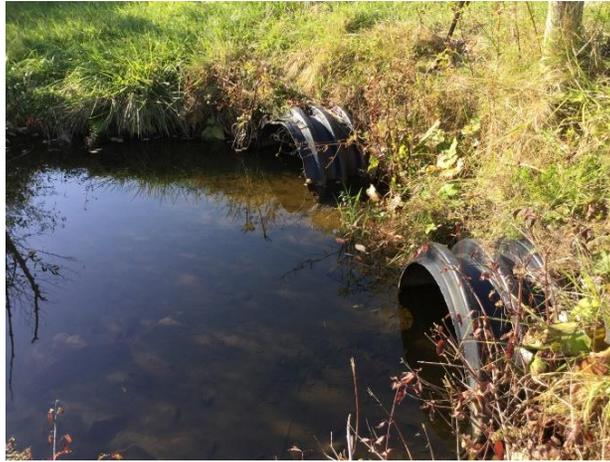
*Figure 10. Two culverts on Sleepy Hollow Road experience flooding during heavy rain events.*
