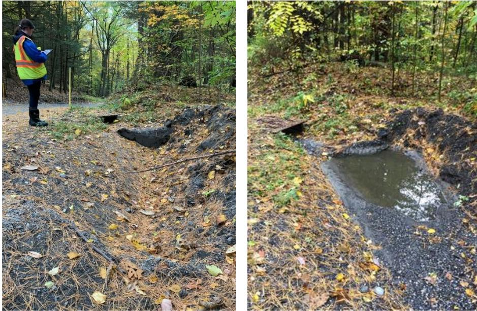
*Figure 11. Pre-rainfall (left) and post-rainfall (right) show ponding in front of the first drop inlet in a series at a high point on Pixley Hill Road in West Stockbridge.*
