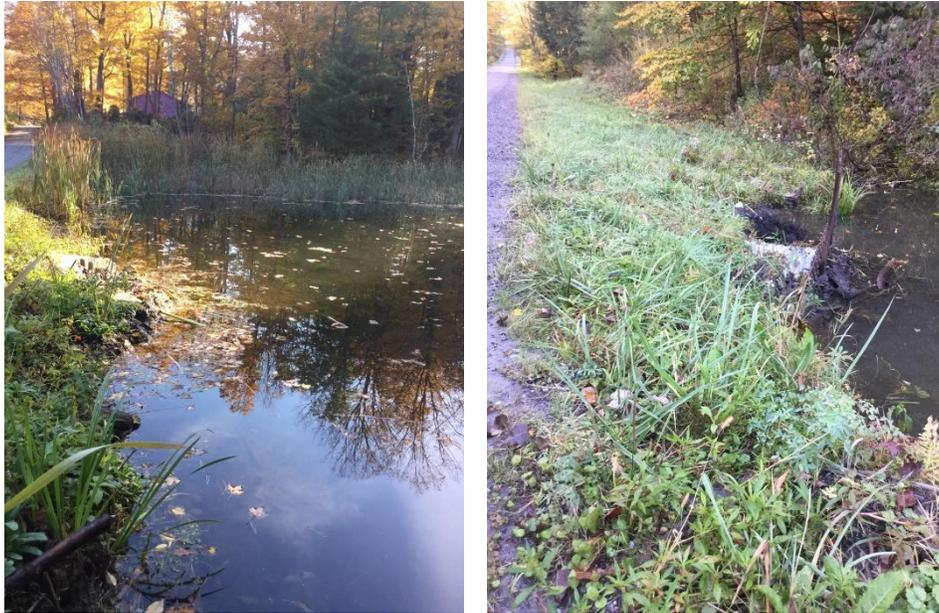
*Figure 10. Road-stream crossing culverts clogs by beavers along West Alford Road. WS.PA-8 (left) has an impoundment behind it. WS.PA-9 (right) has a small impoundment between it and a large beaver dam.*
